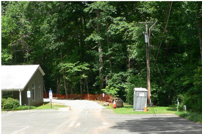
Installing temporary road, giving heavy equipment access to construction site
