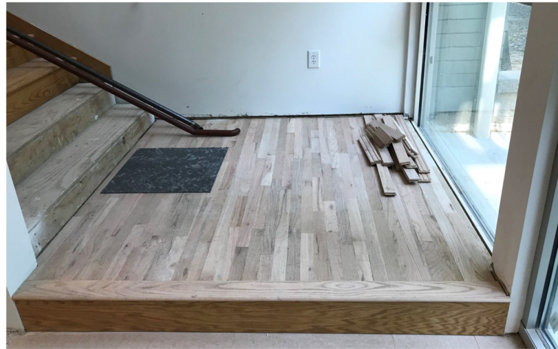
Landing at foot of Stairway to Lower Level
