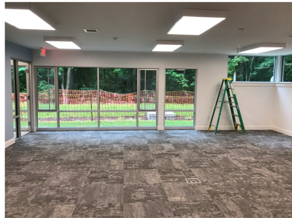
In Living Room on lower level Looking toward south wall (entrance door in far left corner)
