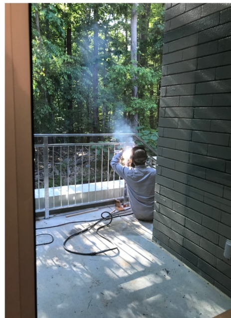
Welder at work: Railing for back porch
