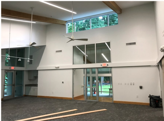
In Gathering Room (Looking toward north wall with main entrance)
