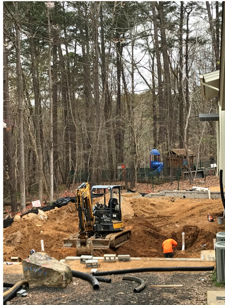
View from old South playground of "rain garden" under construction,
