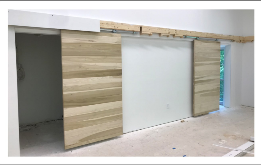
Sliding barn doors for AV and furniture storage spaces in Gathering Room
