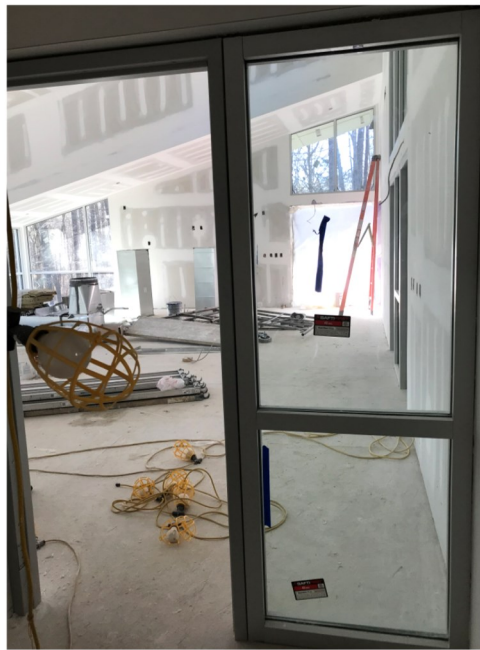
East doorway to Multi-Purpose Room
