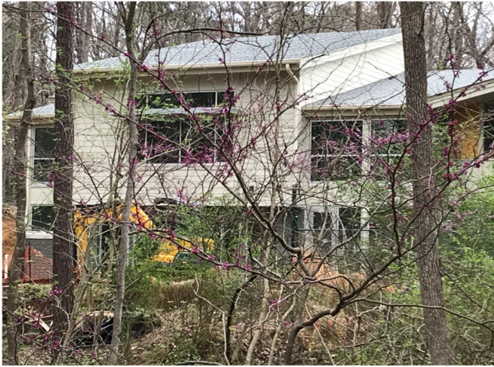
View of new South side from across ravine out back
