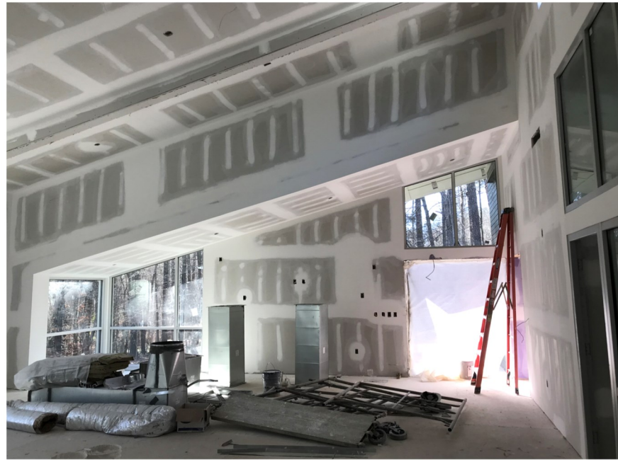
View from just inside East doorway to Multi-Purpose Room
