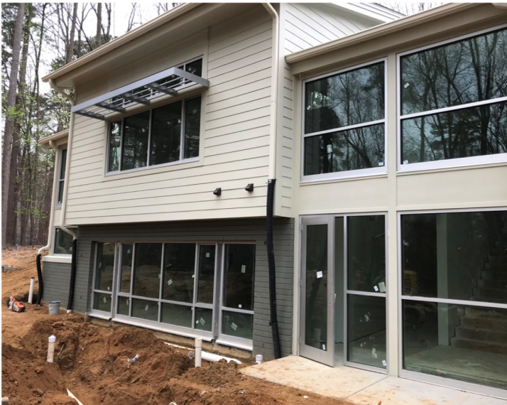
View of South side from edge of "rain garden" under construction
